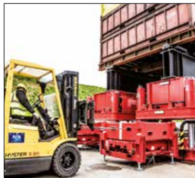
▼ A load is lifted in increments as barrels are slid into the system, lifted, and stacked; forming 'lifting towers'.
