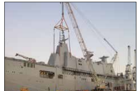
Synchronous hoisting and load positioning
